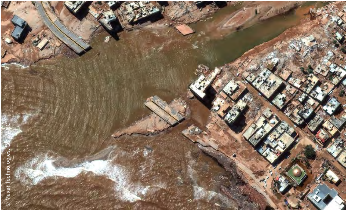
Satellite image of coastal road after floods in Derna, Libya on September 13, 2023.
